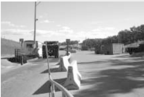
Bourne Integrated Solid Waste Management Facility
