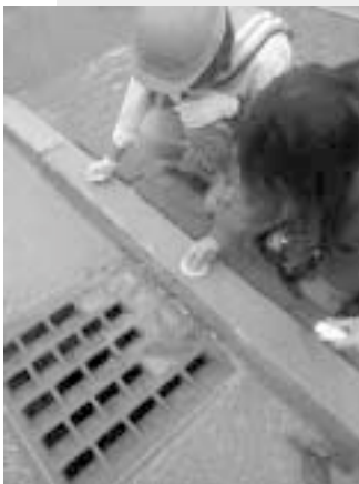
Installing storm-drain markers in Barnstable
