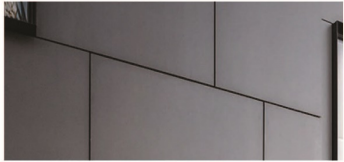
ACM METAL PANEL
